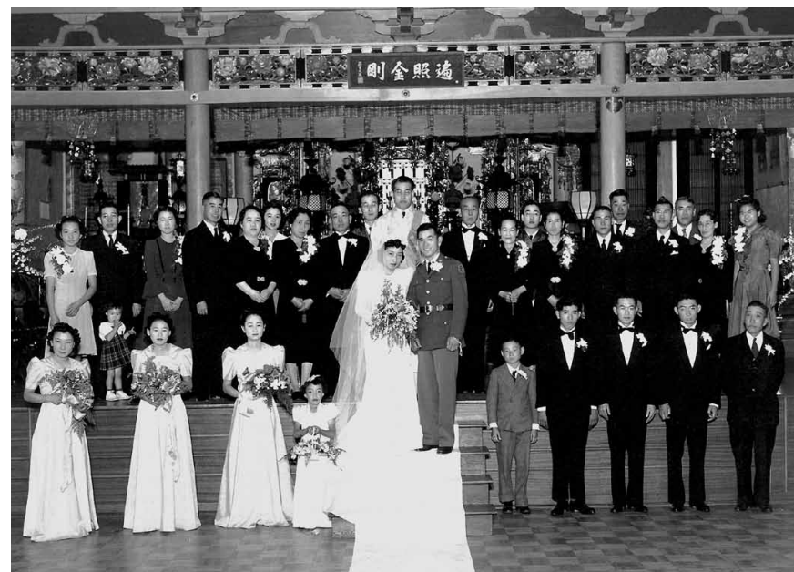
In 1941, Kiyomi and Tsuyoshi Akazawa are the first couple to be married after the completion of the temple construction.
