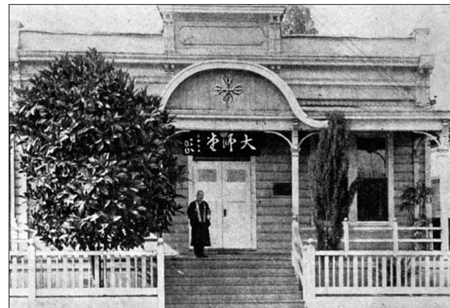
Bishop Shutai Aoyama stands next to a Moreton Bay Fig tree that will be recognized as a living landmark by the City of Los Angeles in 2008.
